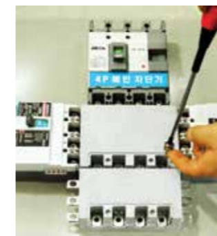
05. Connect Speedbar Block
